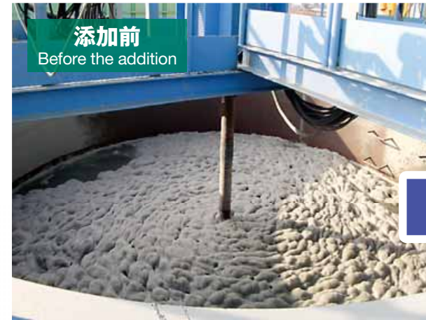
気泡シールド工法の掘削土流体輸送での FT-01 消泡効果(調整槽) Defoaming effect of FT-01 in the Regulation Tank for Hydraulic Transport System
